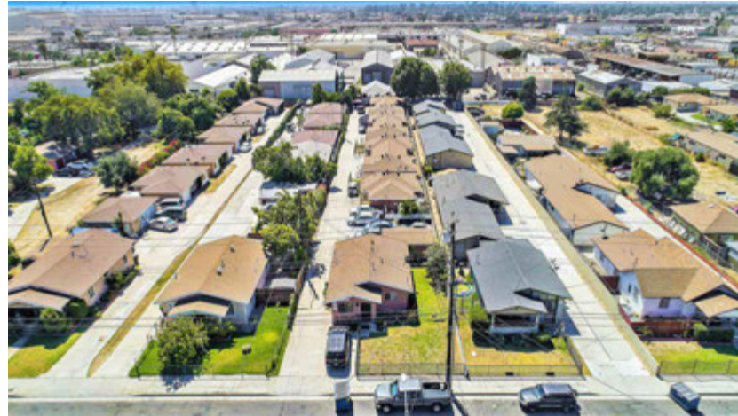
Aerial view in Cudahy showing typical driveway configuration
